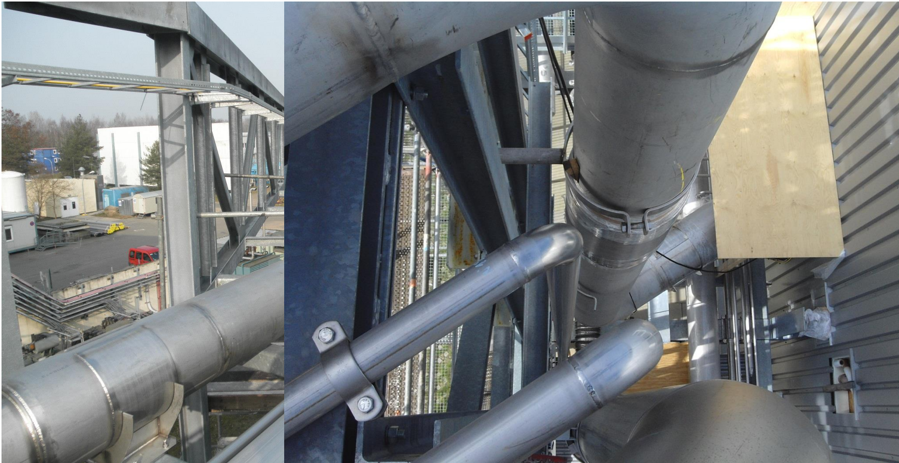
Installation of the XATL1 modules on the piping bridge
