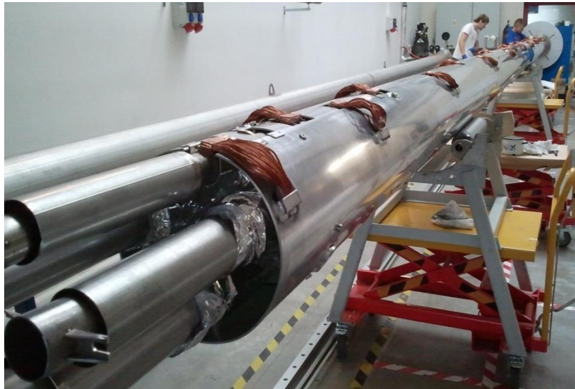
Installation of the process lines in their thermal shield and (courtesy Kriosystem)
