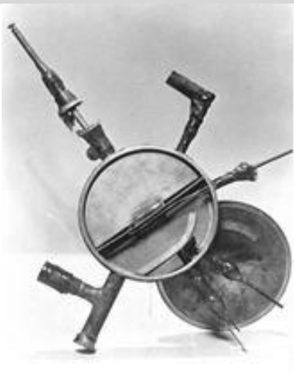
Diagram of the first successful cyclotron constructed by Lawrence and M. S. Livingston. The single dee is five inches in diameter.
